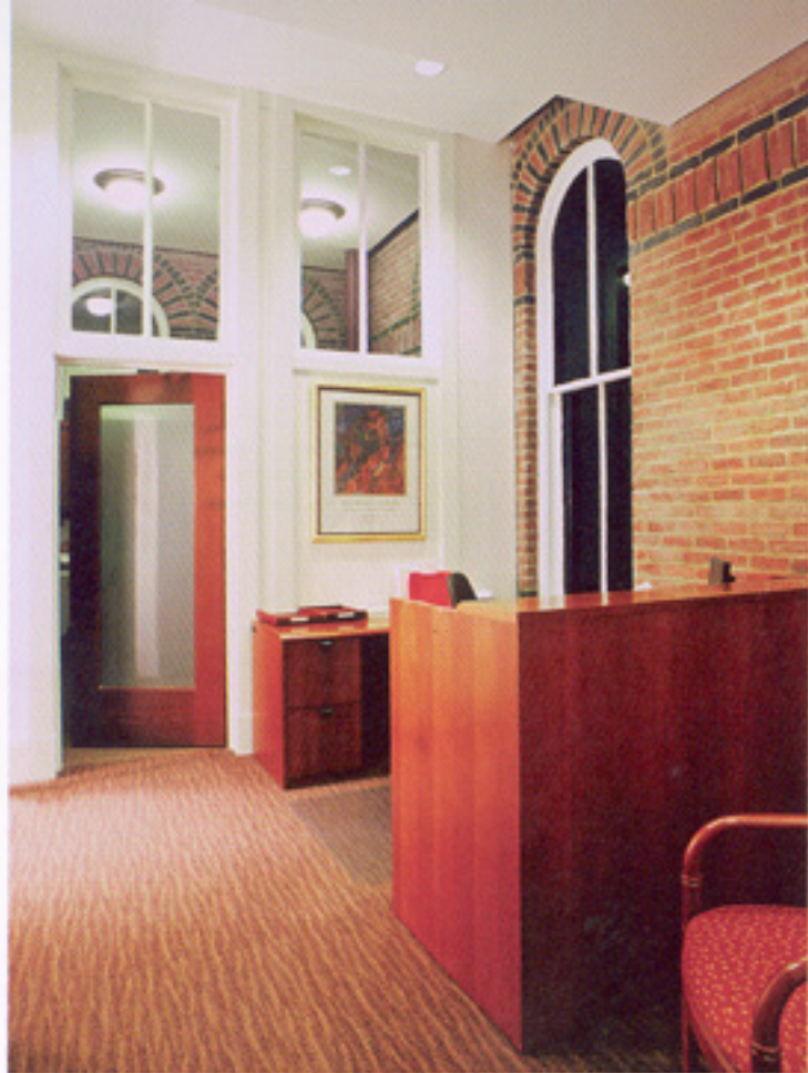
ABOVE LEFT: The original windows and brick façades in the rear of Rockefeller Hall were preserved, creating a unique interior office space in the new infill wing. Photograph by Menefee+Winer
